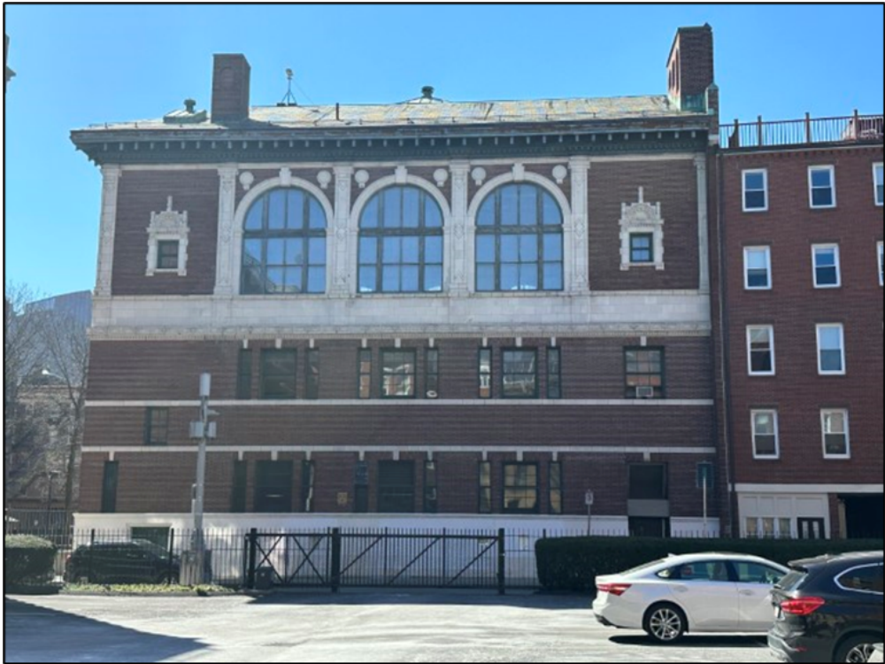
Figure 10. View of northeast elevation at North Bennet Street.
