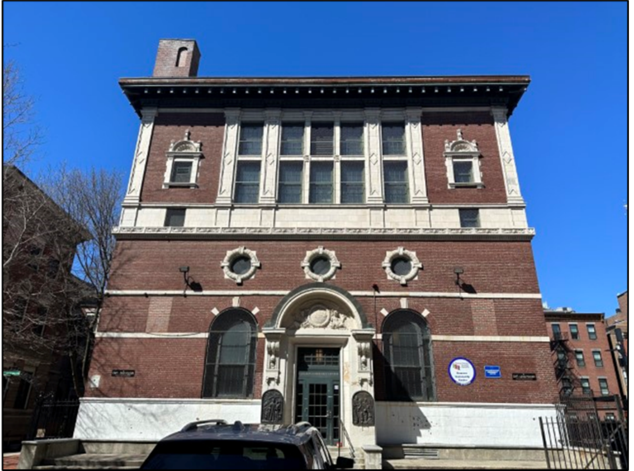
Figure 2. Façade of the Nazzaro Community Center.
