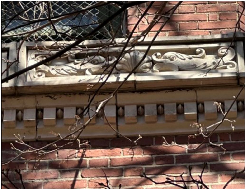
Figure 20. Detail of park-side elevation frieze.
