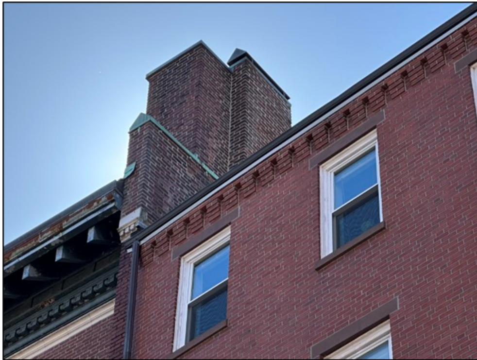
Figure 16. Chimney, cornice, and brick dentil elements.
