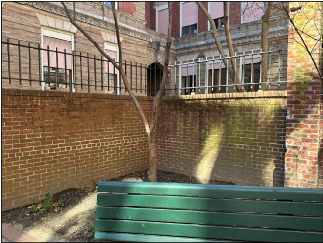
Figure 26. Brick wall, park-side elevation.
