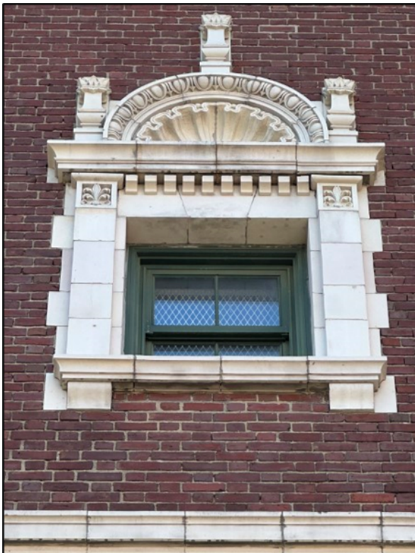
Figure 14. Third-story window on North Bennet Street elevation.
