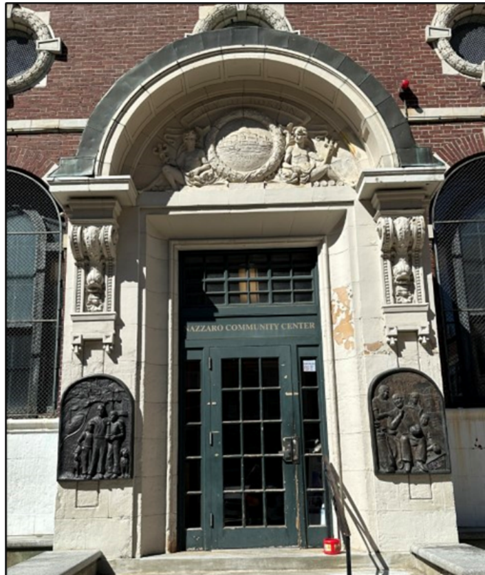
Figure 4. Closeup of front entrance.
