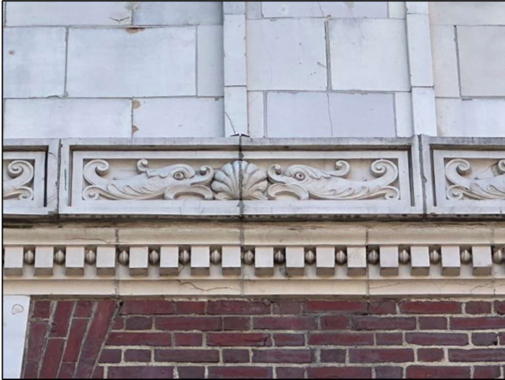
Figure 15. Detail of frieze, North Bennet Street elevation.
