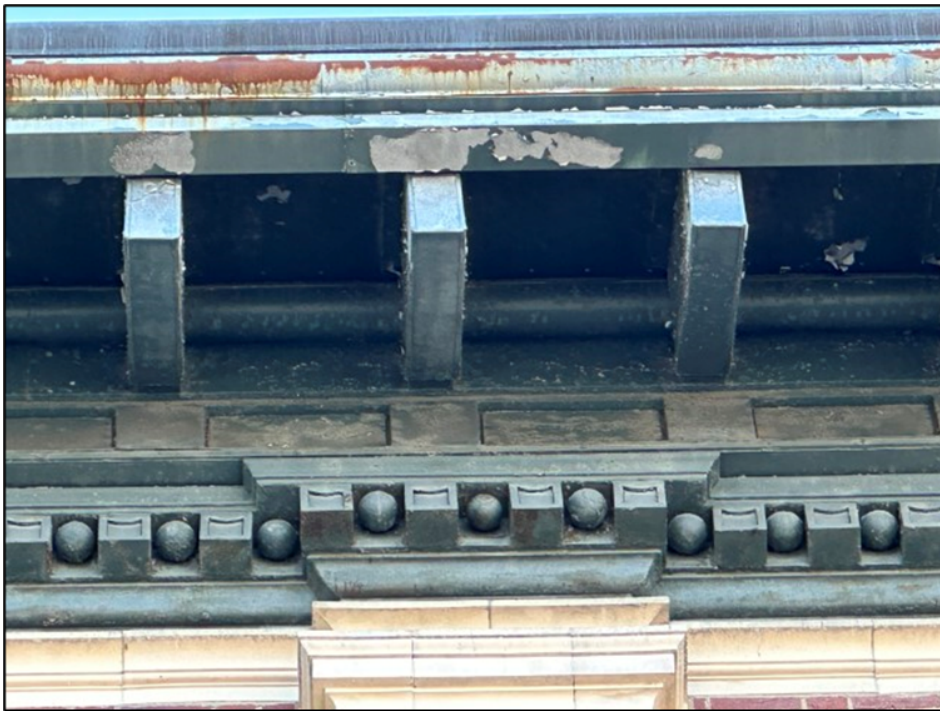
Figure 13. Detail of cornice, North Bennet Street elevation.
