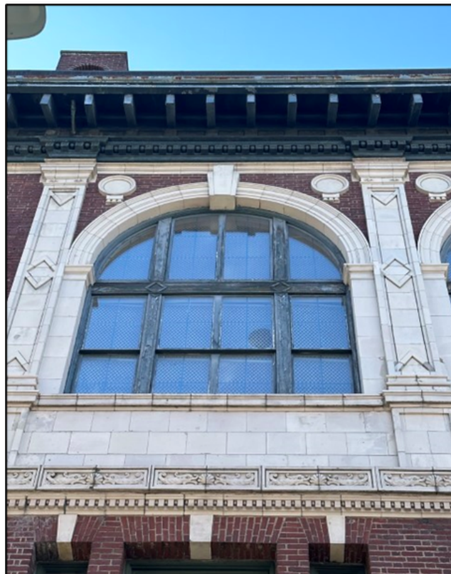
Figure 12. Detail of North Bennet Street elevation rounded arch.
