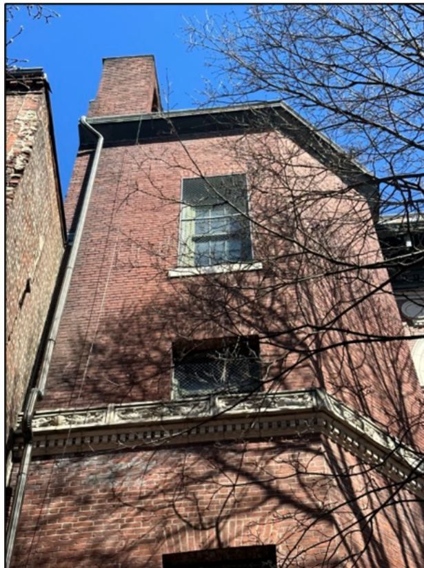
Figure 24. Tower and chimney at park-side elevation.
